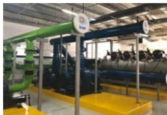
The Kaer Water plant serves the 24-hour, mission-critical requirements of the facility.
