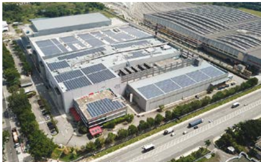
The 3M Rooftop Solar Farm is capable of generating an average of 2,400 MWh of electricity yearly.
