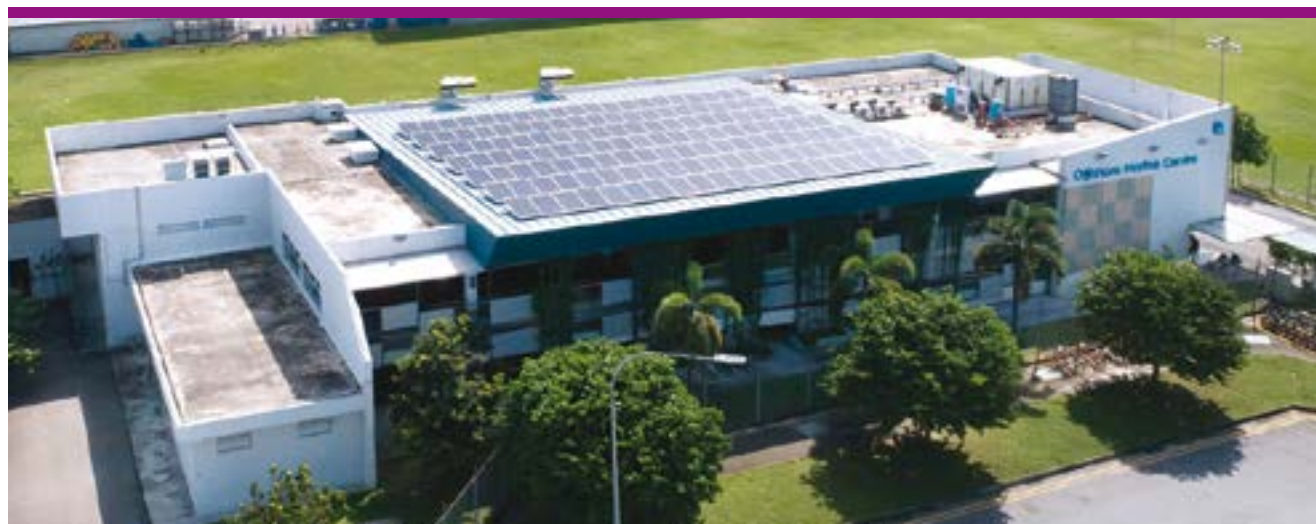
Aerial view of the solar panels on the rooftop of JTC's Offshore Marine Centre.
