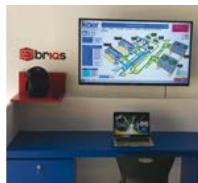
Kaer's control centre with remote monitoring, control and AI capabilities.
