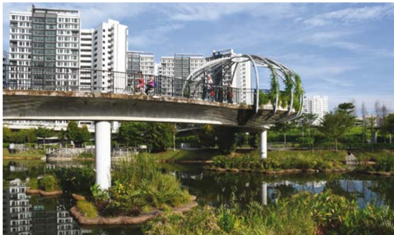
Floating wetland system at My Waterway@Punggol
