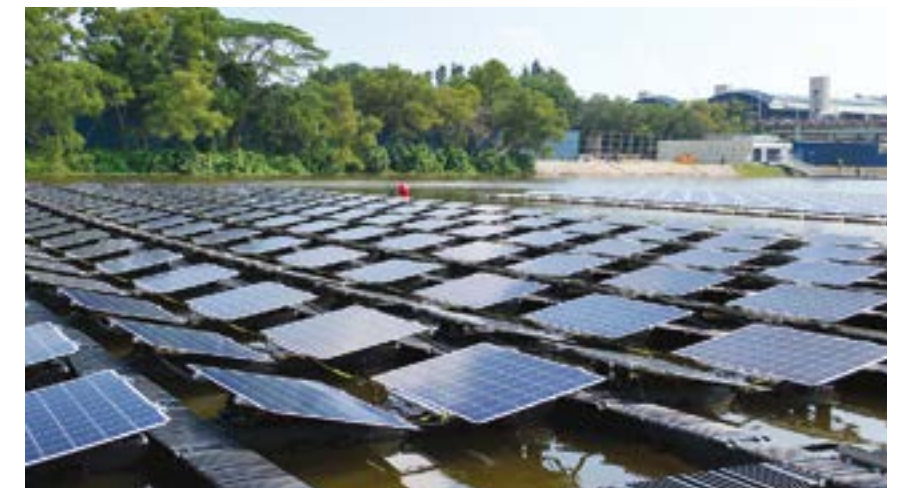
HDB's floating solar system has been deployed at Tengeh Reservoir.
