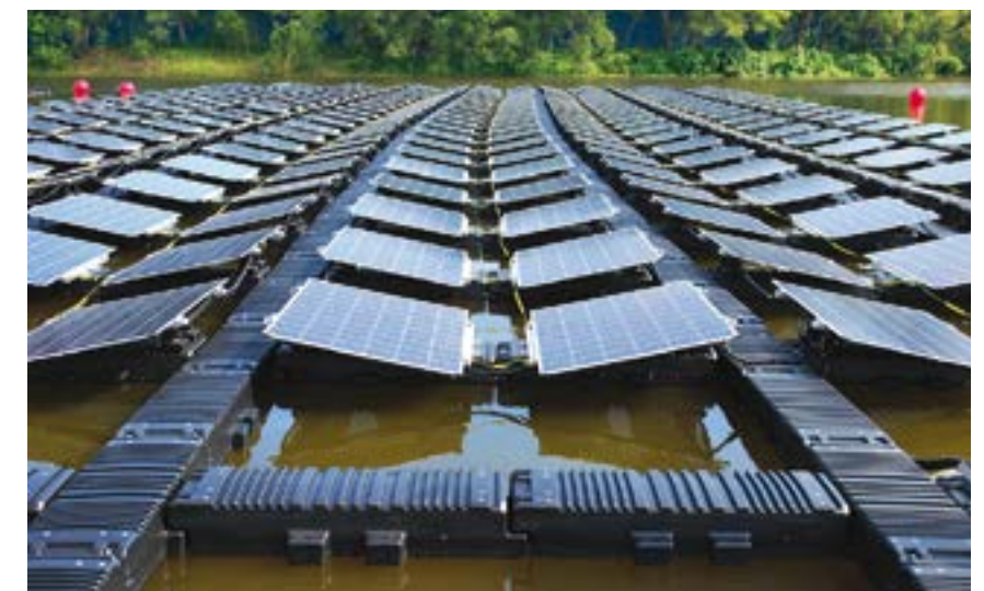
Each maintenance pathway is designed to serve two rows of solar panels, reducing the need for additional maintenance pathways.
